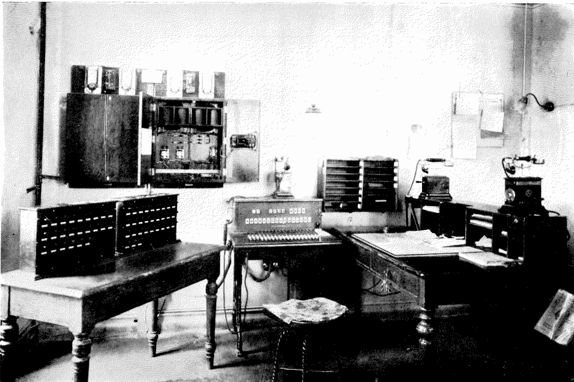
Figure 13—Telephone Train Dispatching—Goteborg Dispatching Office, Sweden
