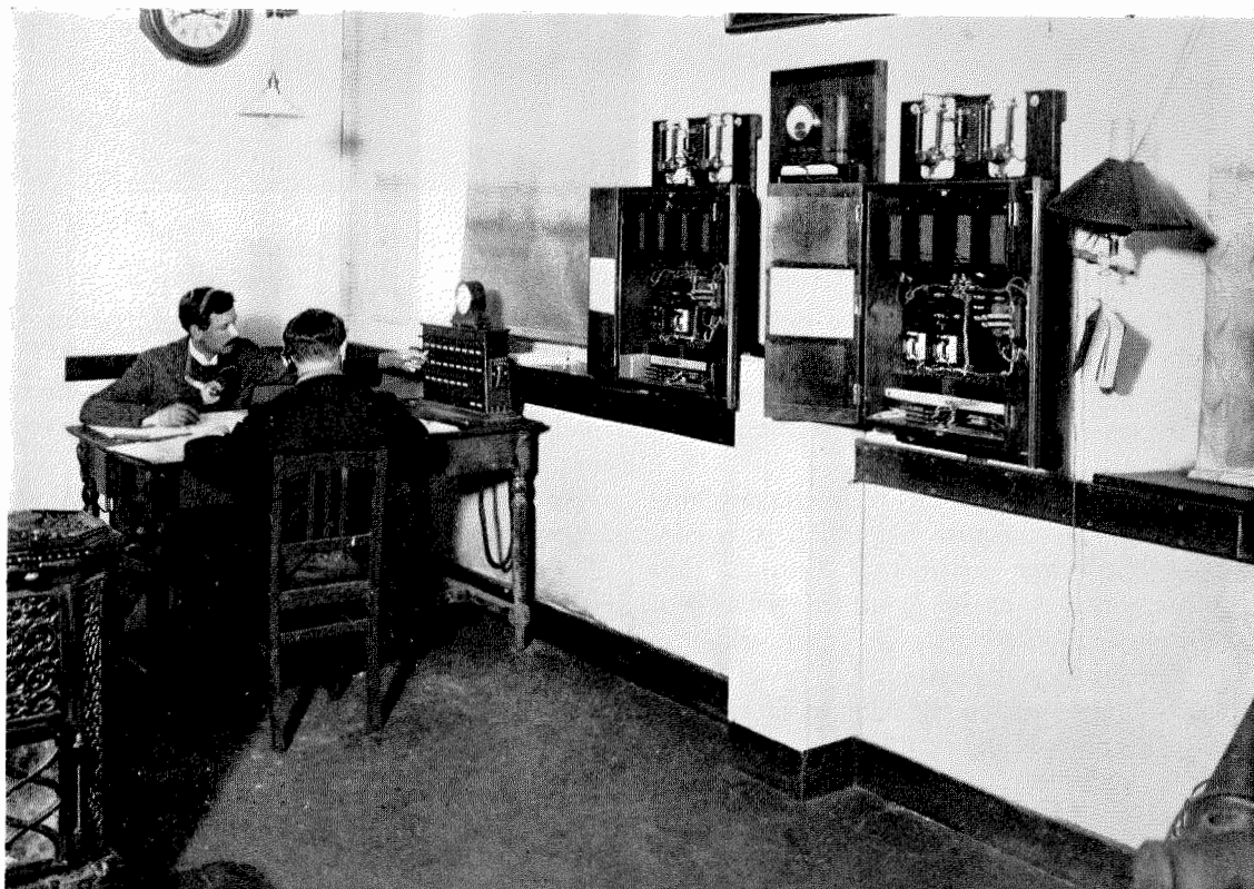
Figure 11—Dispatcher's Office—Bruxelles Nord, Belgium
